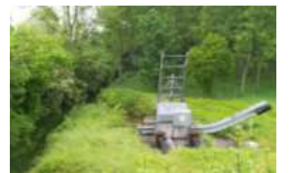
Upgrading Pumping Station
